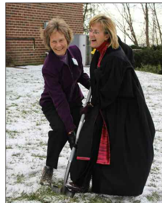
Board of Trustees Chair Joan Darrah and Rev. Kate Walker break ground for Mt. Vernon Unitarian Church's new solar-geothermal system.
